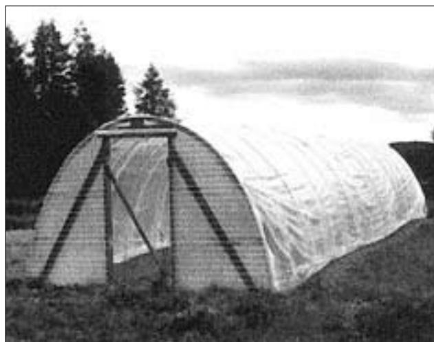
Figure 1. Portable field hoophouse, 10’ wide by 42’ long, resting directly on soil surface in the field.
